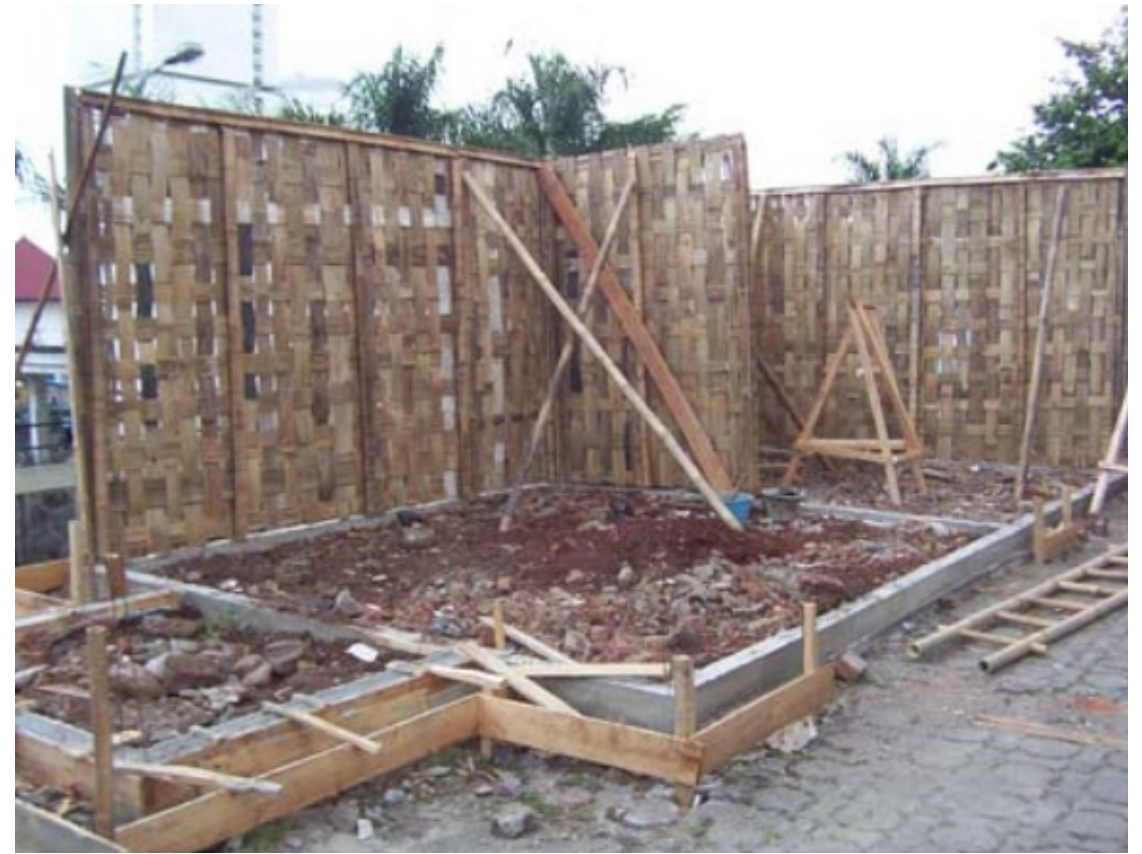
Bamboo Panel Erection
