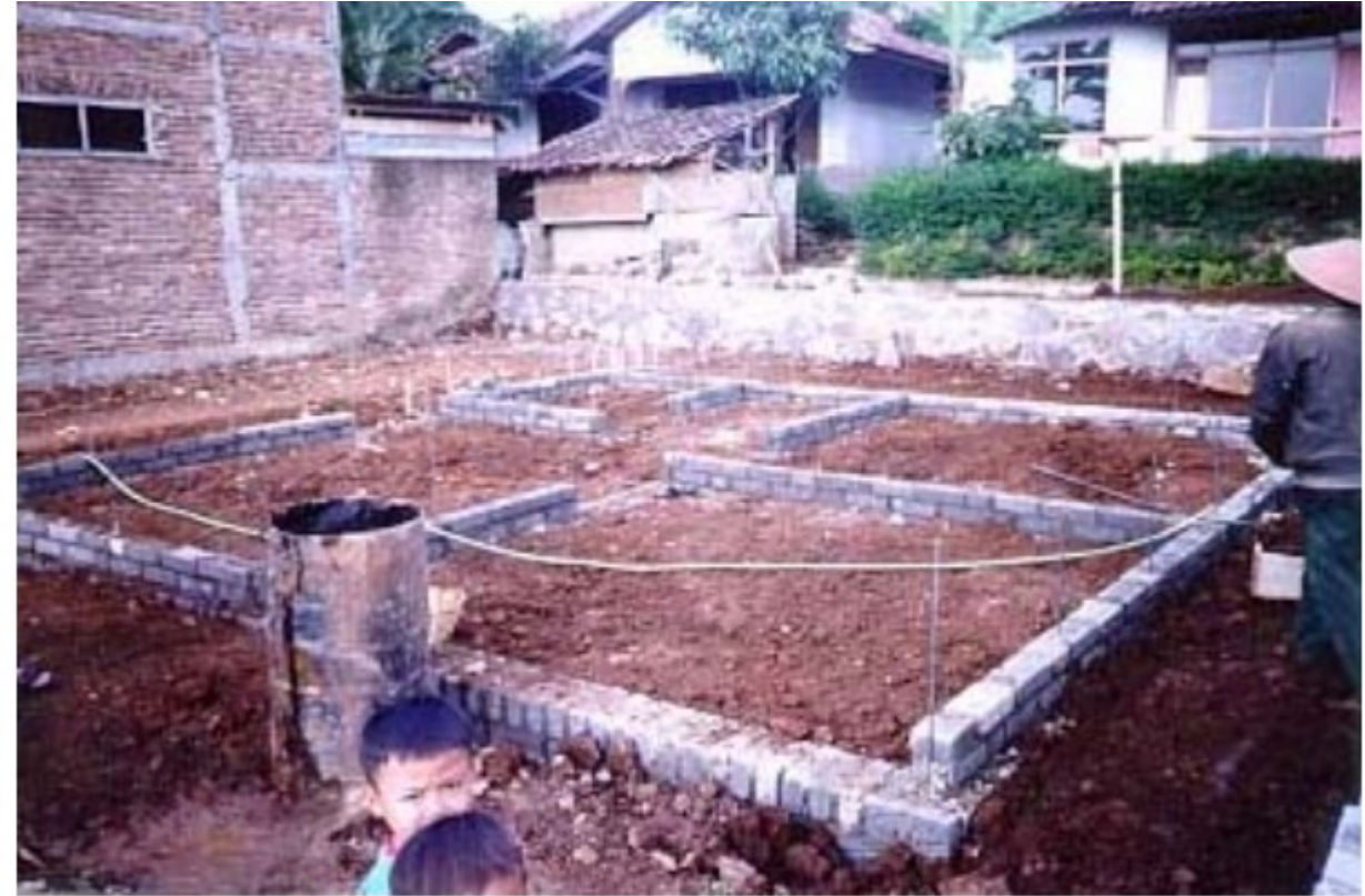
Step 2 : Land preparation and tie beam construction on site, in the same time with bamboo workshop
