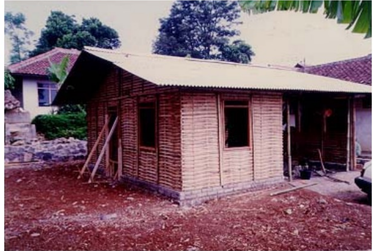
Step 3 : Erecting the prefabricated bamboo panel and constructing roof
