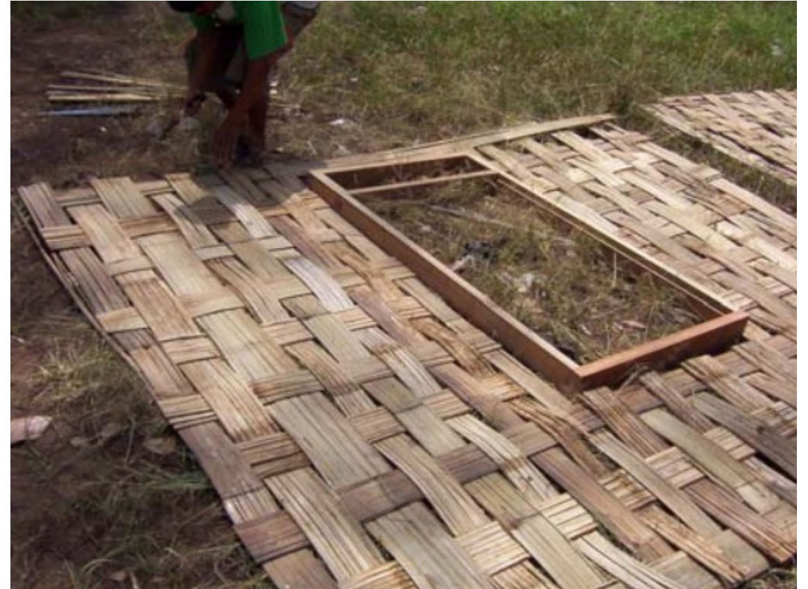
Bamboo Panel Prefabrication
