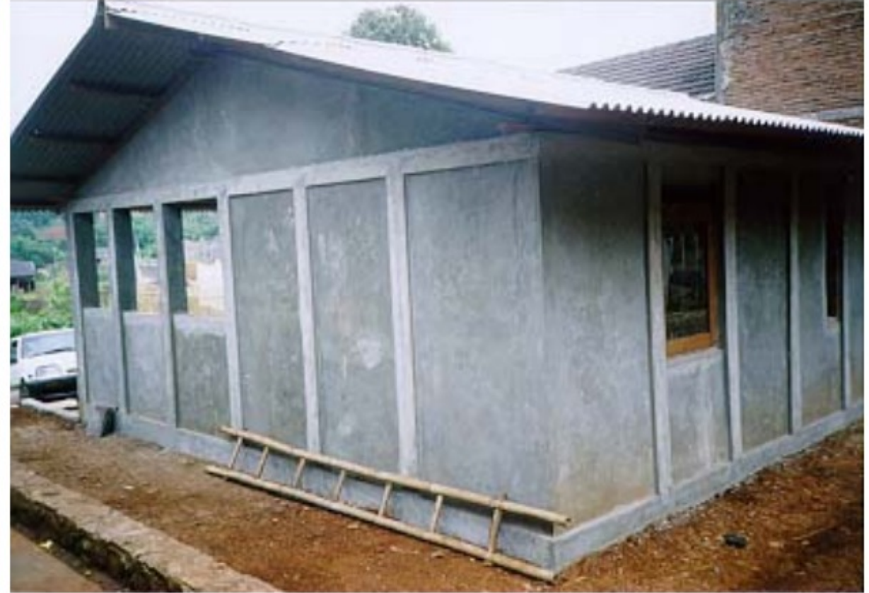
Step 4 : Plastering bamboo house to become ‘permanent house’
