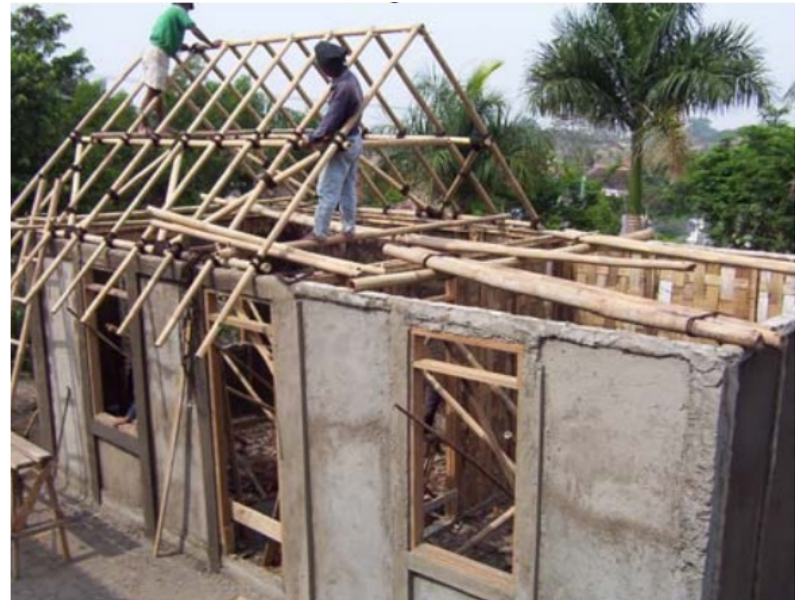
Plastering Process and Roof Construction
