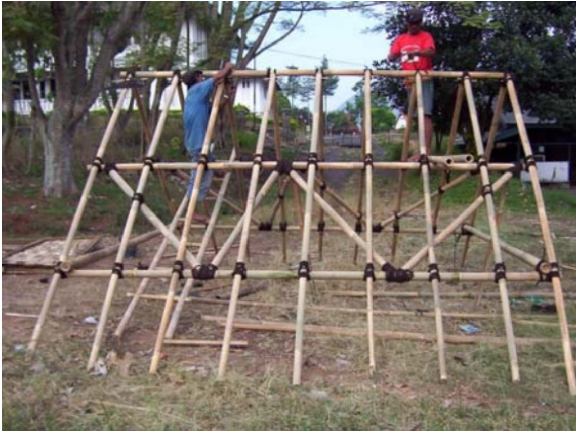
Roof Frame Prefabrication
