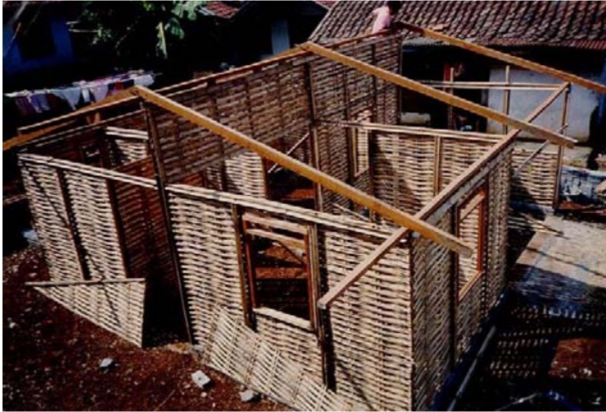
Step 3 : Erecting the prefabricated bamboo panel and constructing roof
