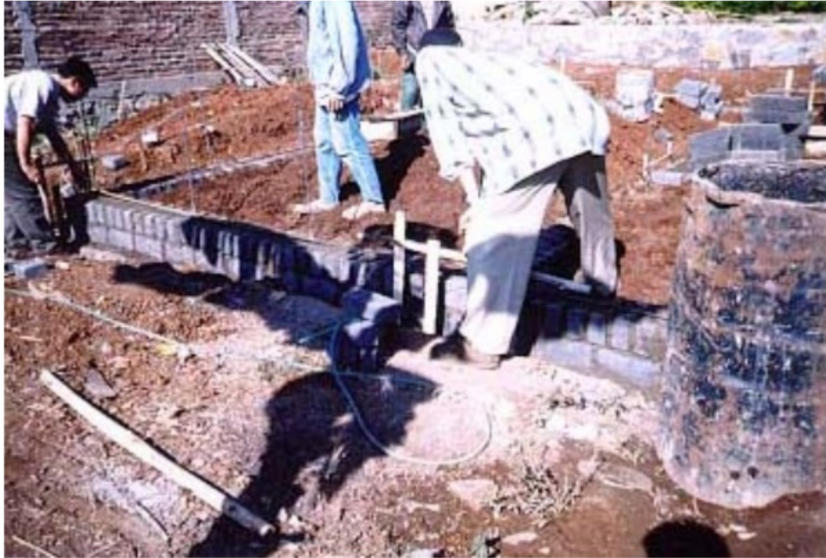
Step 2 : Land preparation and tie beam construction on site, in the same time with bamboo workshop
