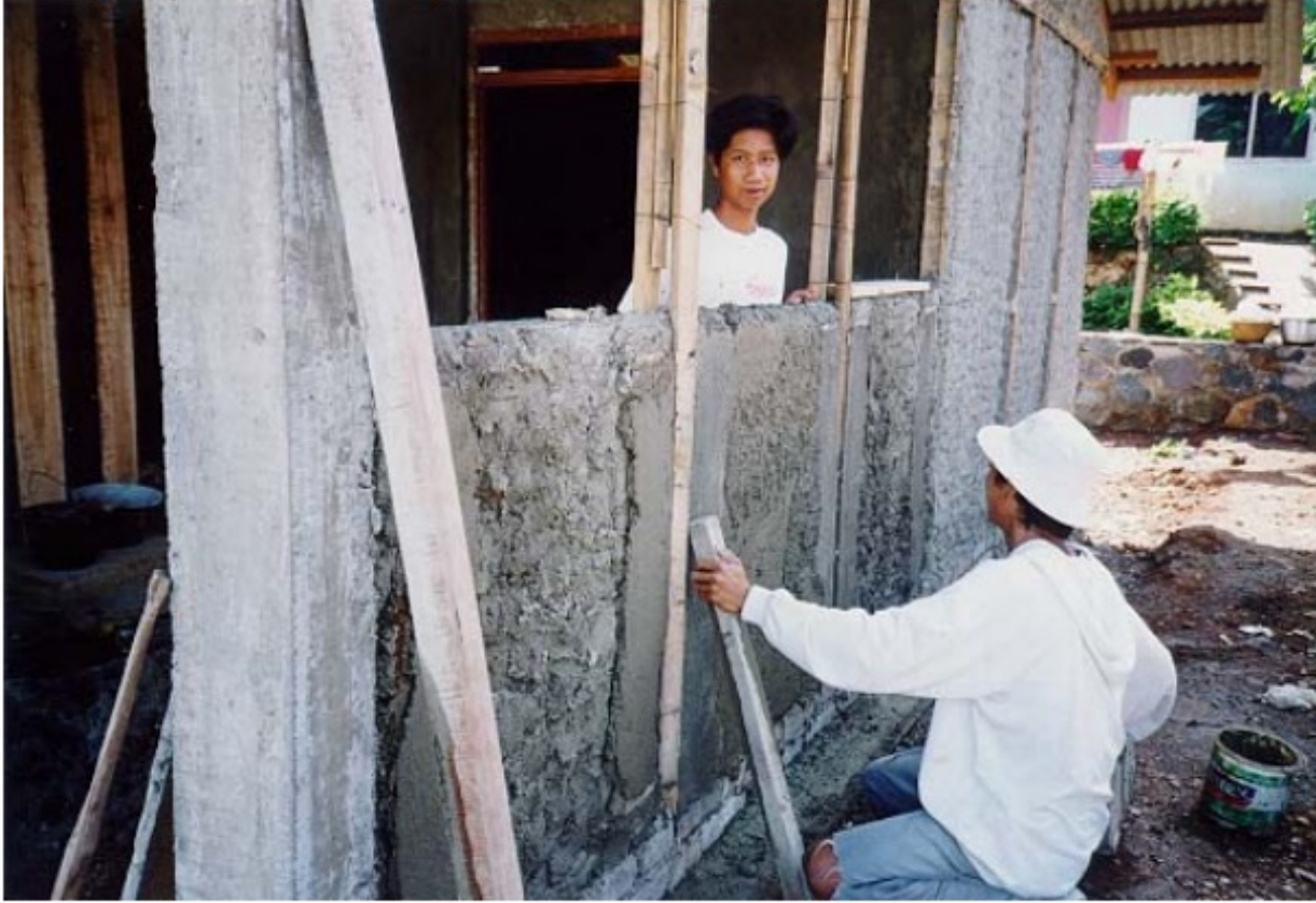
Step 4 : Plastering bamboo house to become ‘permanent house’
