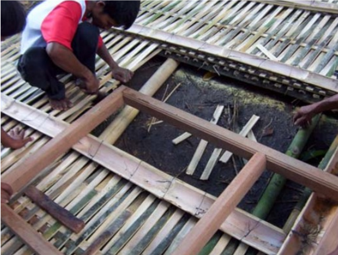
Bamboo Panel Prefabrication
