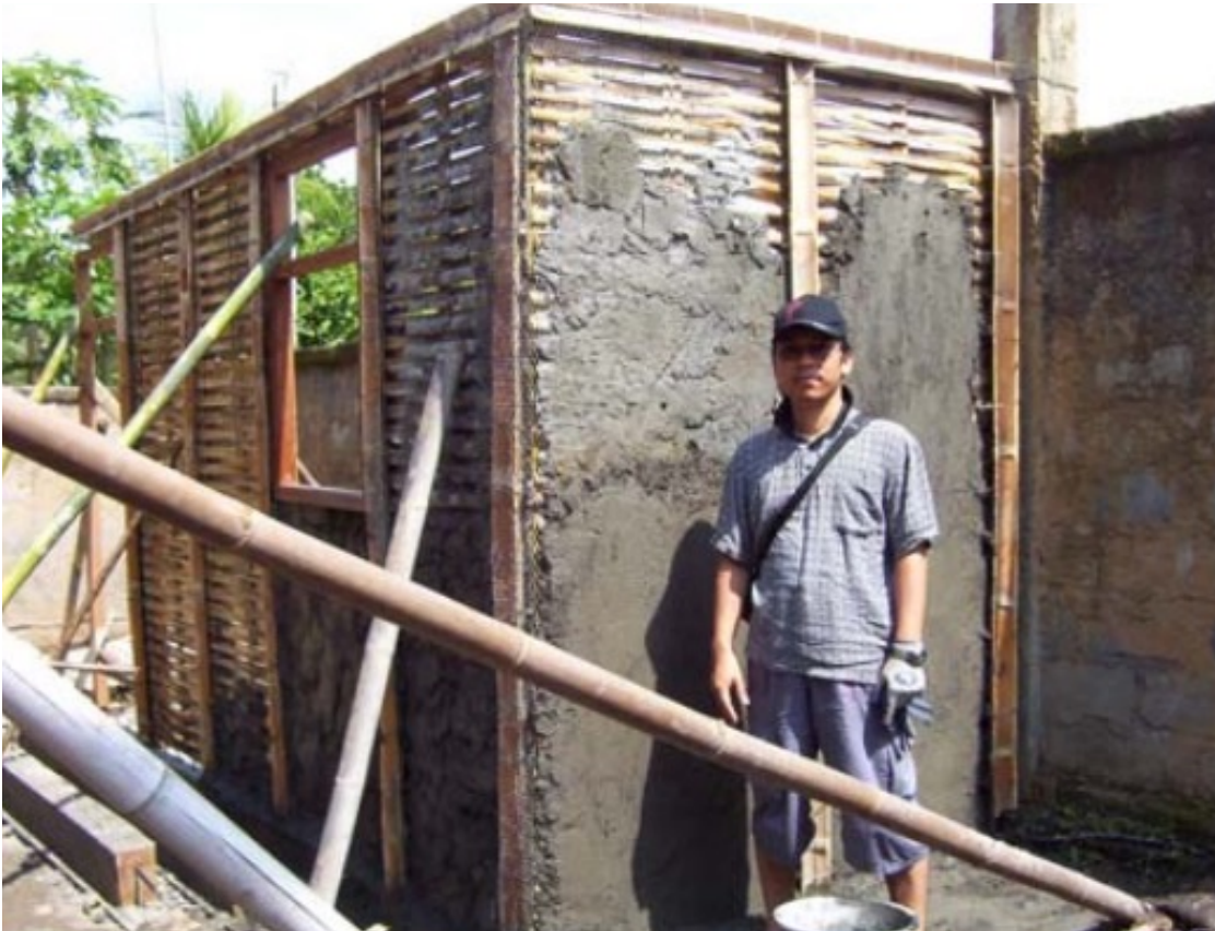
Plastering the Bamboo Wall
